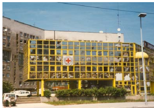
Damaged Red Cross Building (Photo: J. Riggs)
