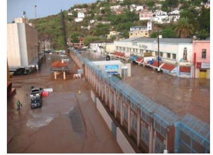
Wall-induced floods devastate Nogales, Mexico. Credit: U.S. Customs and Border Protection
